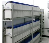
Both ac and station battery voltage sources can be used. If one supply fails, the network will not be affected.
